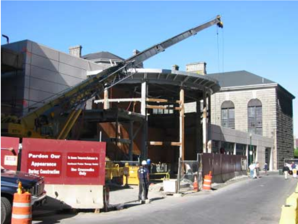
Demolition in progress at NPTC, July 2002.
